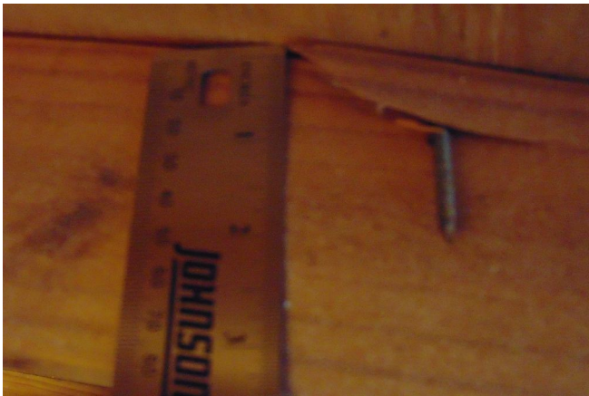
Roof Deck Attachment
