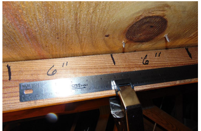
Roof Deck Attachment
